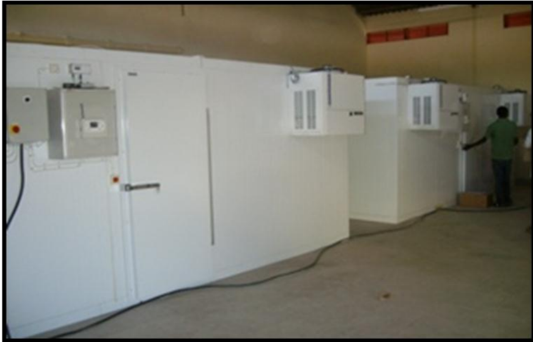
Figure 3: New Cold Room at the National EPI Unit
