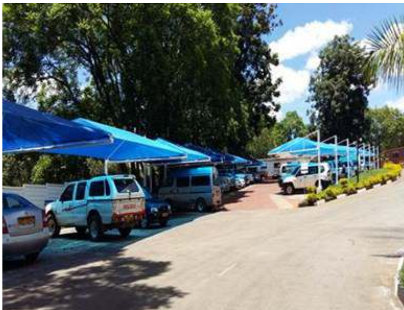
Figure 20 (a) : Parts of the renovated WHO premises at Highlands,
