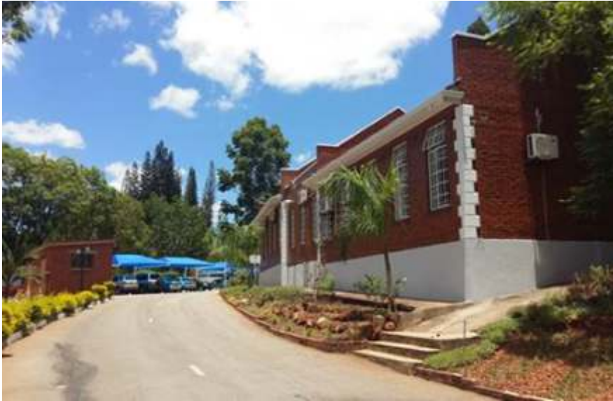
Figure 20 (b) : Parts of the renovated WHO premises at Highlands, Harare
