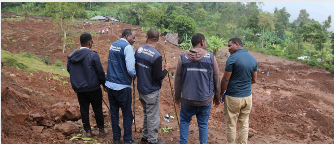
Wide view of the affected area, showcasing the extensive damage and displacement.
